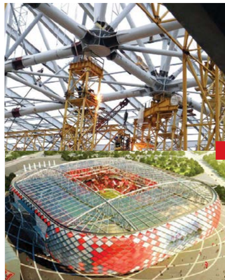
Multipoint system of lifting and lowering roof's frame "Spartak" stadium in Moscow, "Ruby" in Kazan and "Fischt" in Sochi.
