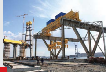
Hydraulic equipment «Enerprom» for construction of the bridge to the island «Russkii» in the Eastern Bosphorus Strait, Vladivostok.
