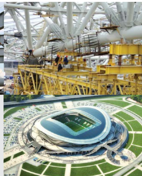
Multipoint system of lifting and lowering roof's frame "Spartak" stadium in Moscow, "Ruby" in Kazan and "Fischt" in Sochi.
