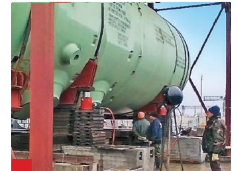
System for simultaneous lifting of the object for assembling the reactor plant of nuclear power station WWER – 1000, Volgogradsk.
