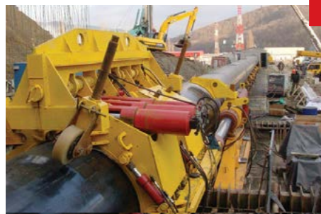
Equipment UPT-700 for pushing pipes in tunnel transition for oil products transportation, Krasnodar region
