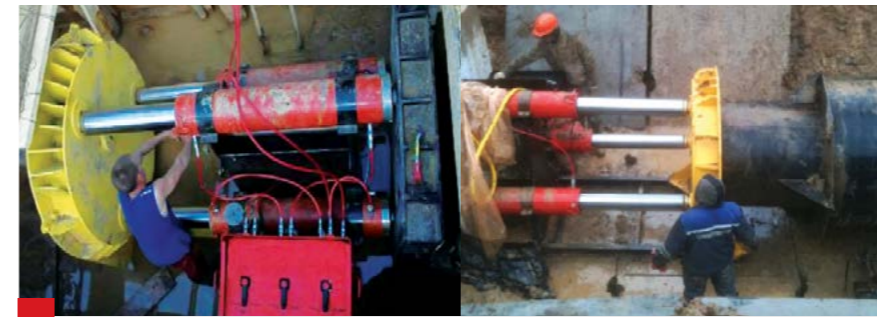
Trenchless pipes laying system UBPT «Horizon» for a governmental project «Oil pipeline «Easten Siberia–Pacific»
